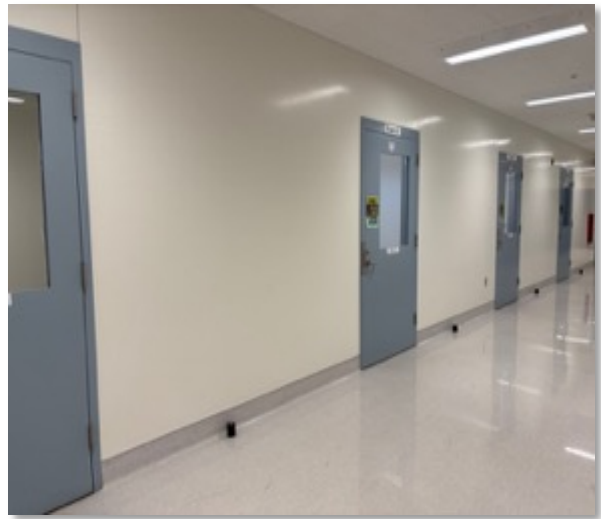
Photo 16. Receiving and Release hallway of PCP exam rooms. Photographed 5-19-2026.
