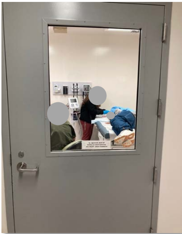
Photo 14. Exam room lacked adequate visual privacy. Photographed 1-5-2026.
