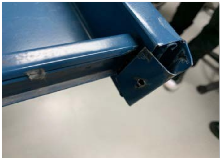
Photo 11. Drawer in disrepair. Photographed 1-5-2026.
