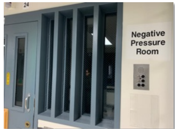
Photo 24. CTC negative pressure room. Photographed 2-20-26.
