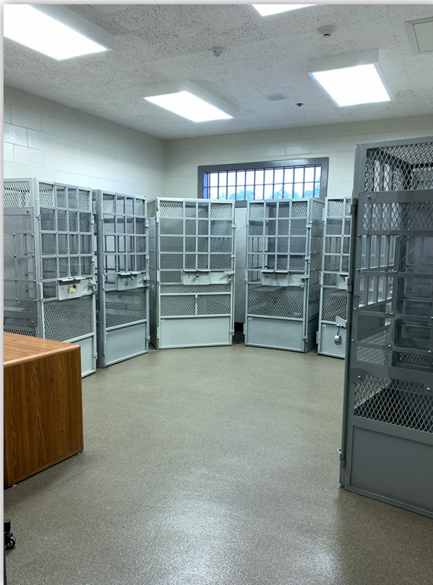
Photo 2. One of Corcoran's mental health group treatment rooms with temporary holding cells used for restricted housing units.
