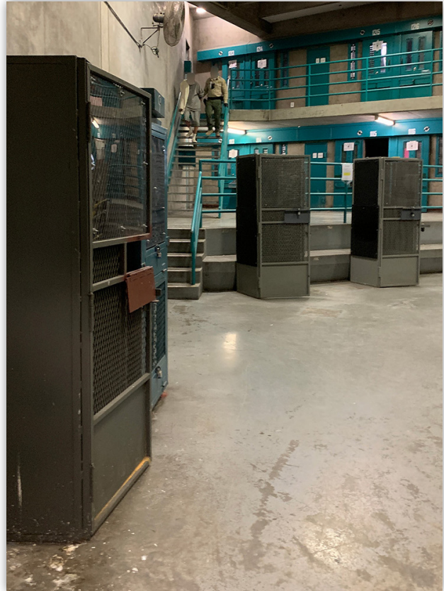
Photo 3. Temporary holding cells at California State Prison, Sacramento.
