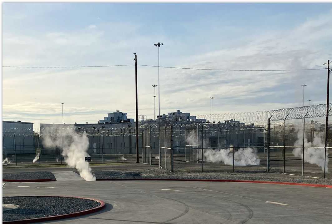
Photo 1. Steam seeping from cracked pipes at California State Prison, Corcoran. Source: OIG audit staff.
