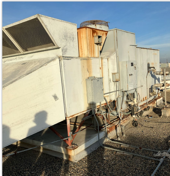
Photo 3. An evaporative cooling system at California State Prison, Corcoran. Source: OIG audit staff.
