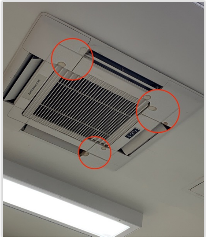
Photo 6. Staff for Madrone medication room reported water leaking from the air conditioning unit when it rains (photographed on 5-11-22).
