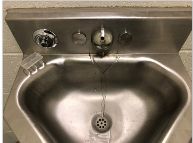
Photo 13. Nonfunctioning sink in patient restroom (photographed on 12-16-21).
