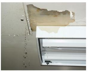
Figure 4 – Water leak in light fixture. Photo: CCWF Plant Operations
